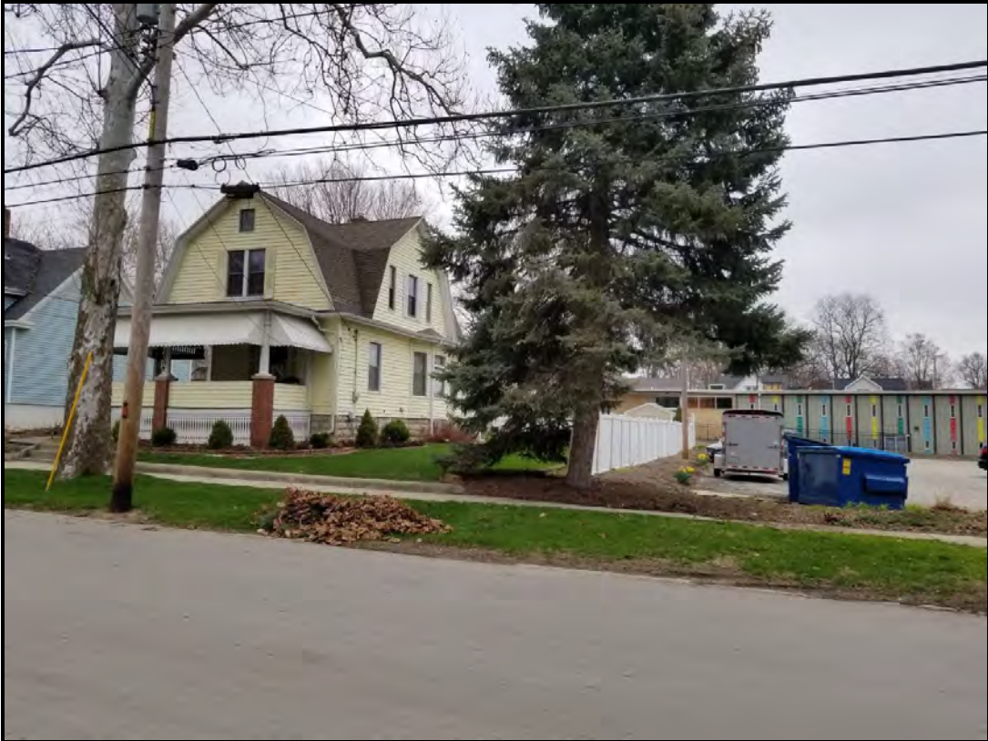
Figure 6 Residence at 1309 N. Lee Street pictured here is proposed to be demolished in phase 2 of the parking lot development.
