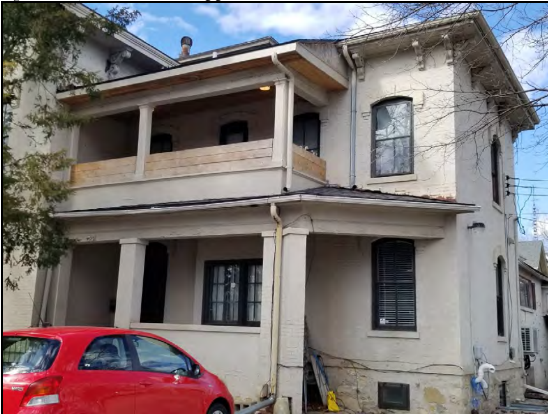
Figure 5 South elevation - notice gutters and downspouts.
