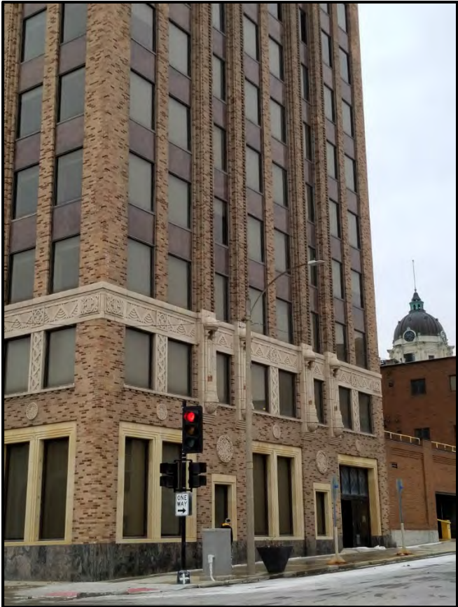
Figure 9 North elevation of the State Farm building.
