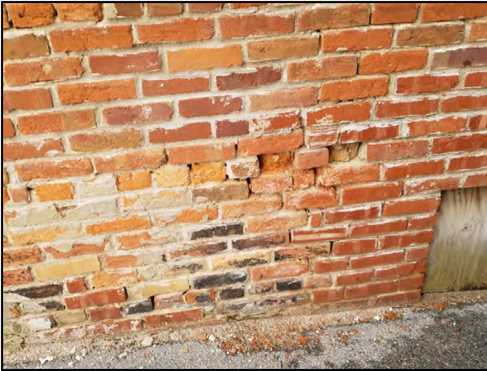
Figure 4 East elevation of the subject property.
