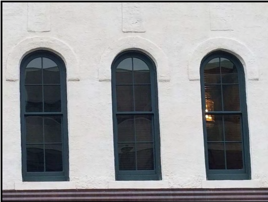
Figure 6 Windows on second floor at 115 W. Front Street.
