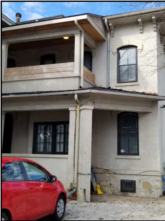
Figure 2 Rear addition - South elevation facing E. Chestnut Street.
