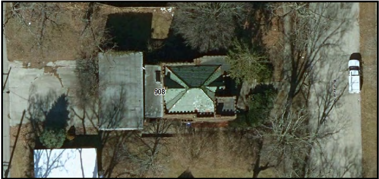
Figure 3 Aerial photo of the roof at the subject property.
