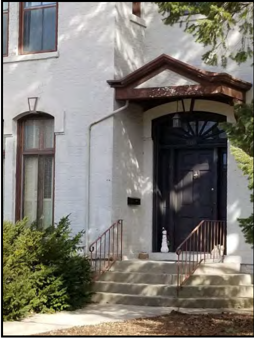
Figure 6 Front door - west elevation facing N. McLean Street.
