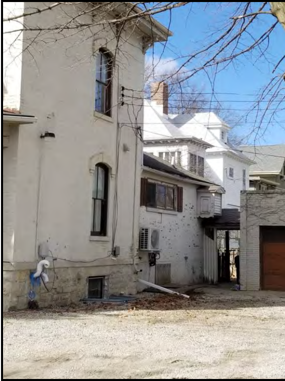
Figure 4 Rear, East elevation showing gutter.
