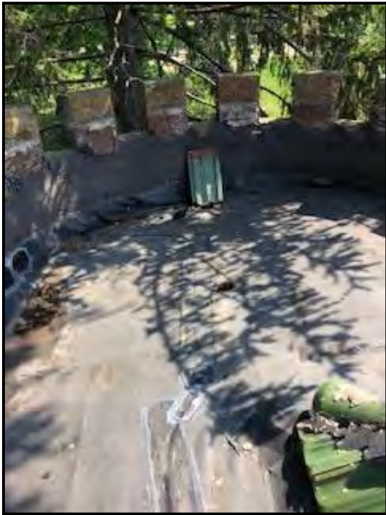
Figure 13 View of the flat portion of the roof.
