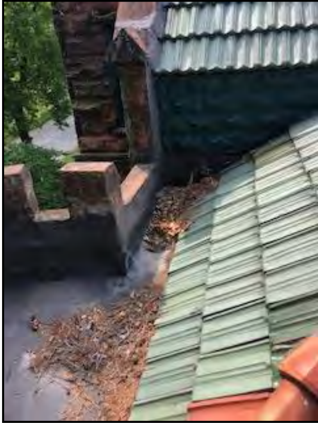
Figure 5 View from on top of roof.
