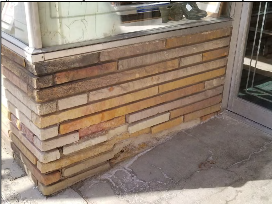
Figure 7 Facade at entrance of the subject property.
