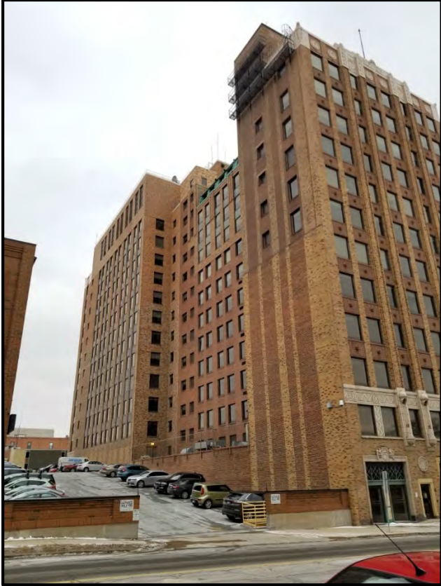
Figure 4 West Elevation of the State Farm building.
