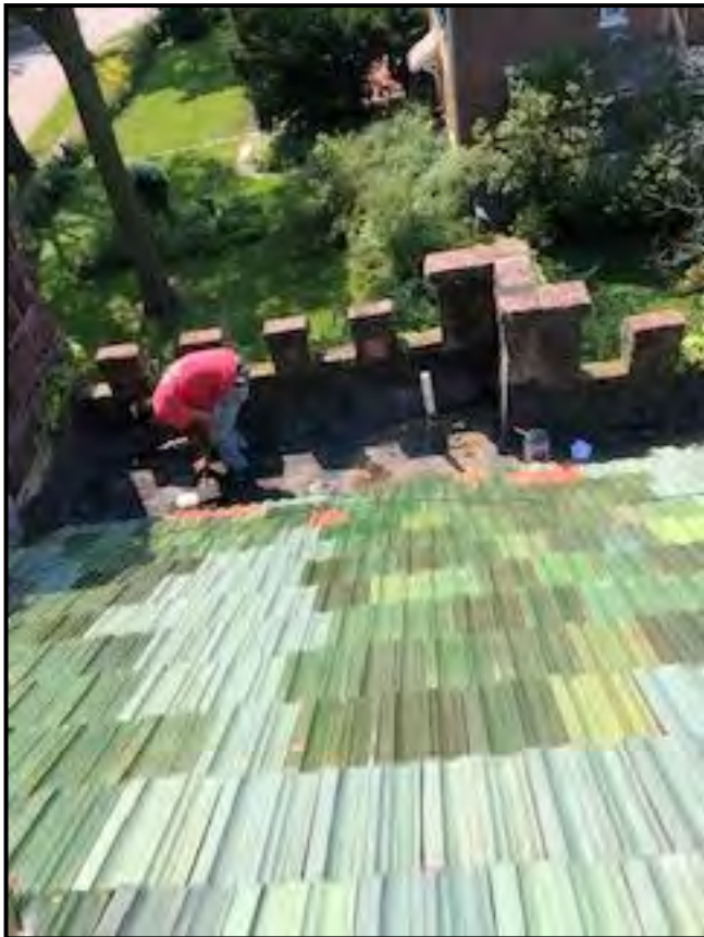
Figure 10 View from top of roof.
