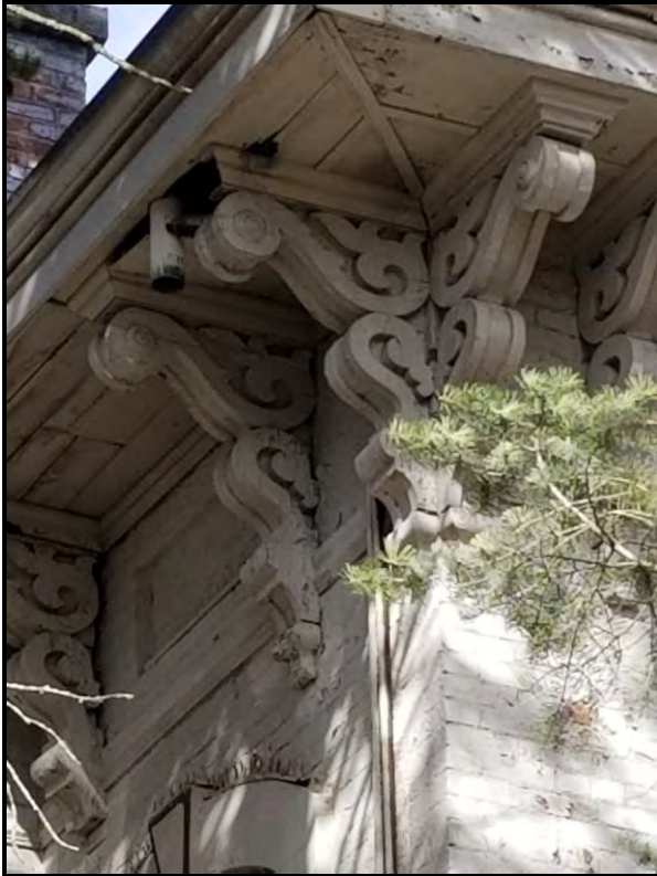
Figure 10 Closeup of downspout shown above on front facade at cornice.
