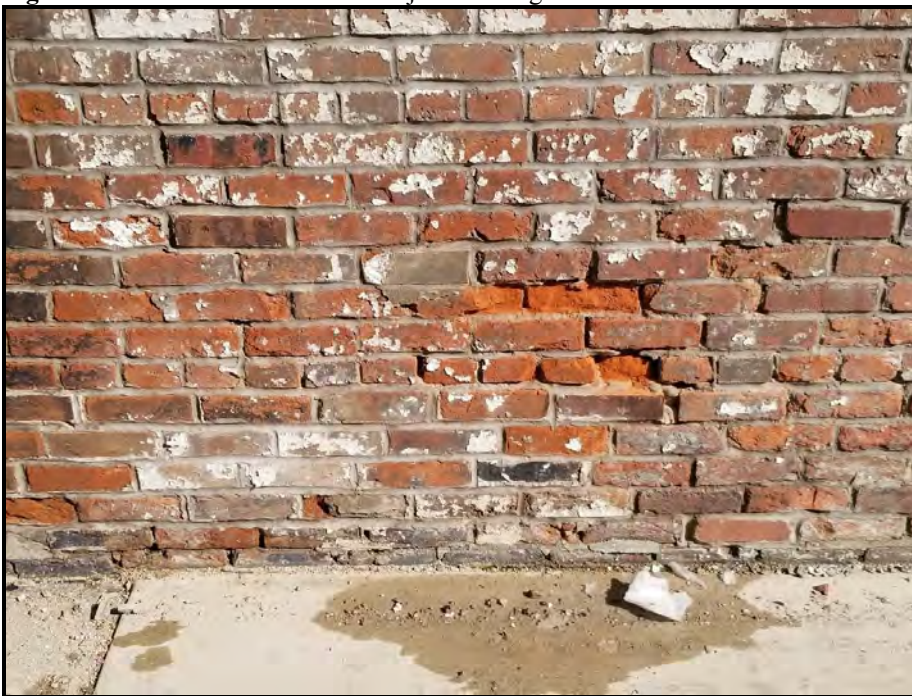
Figure 9 West elevation of the subject property.
