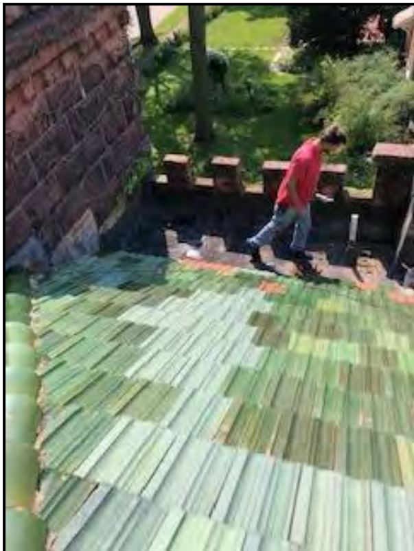
Figure 12 View from top of roof.
