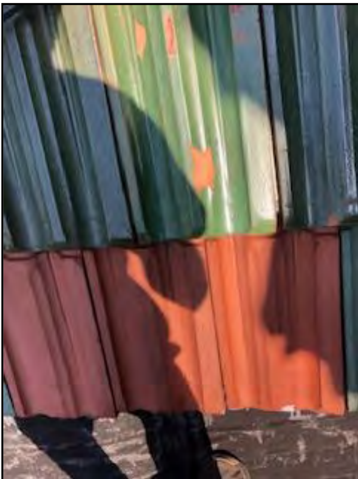
Figure 8 Ceramic roof tiles.
