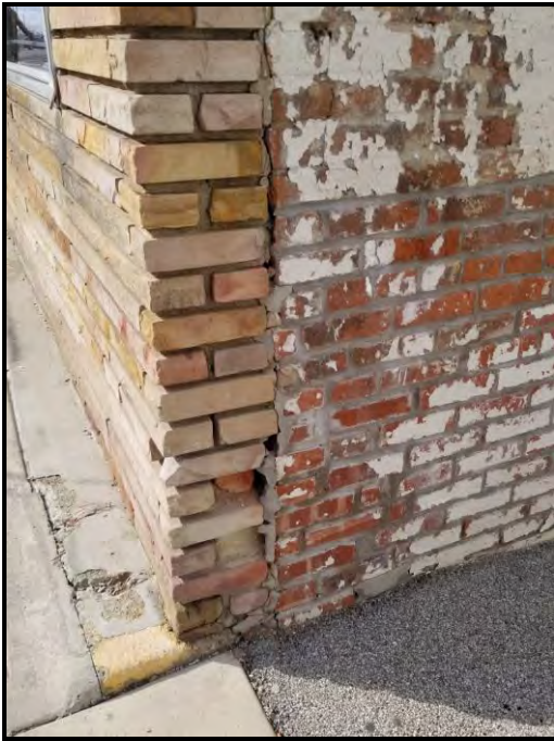
Figure 2 Southeast corner of facade at 107 W. Monroe Street.
