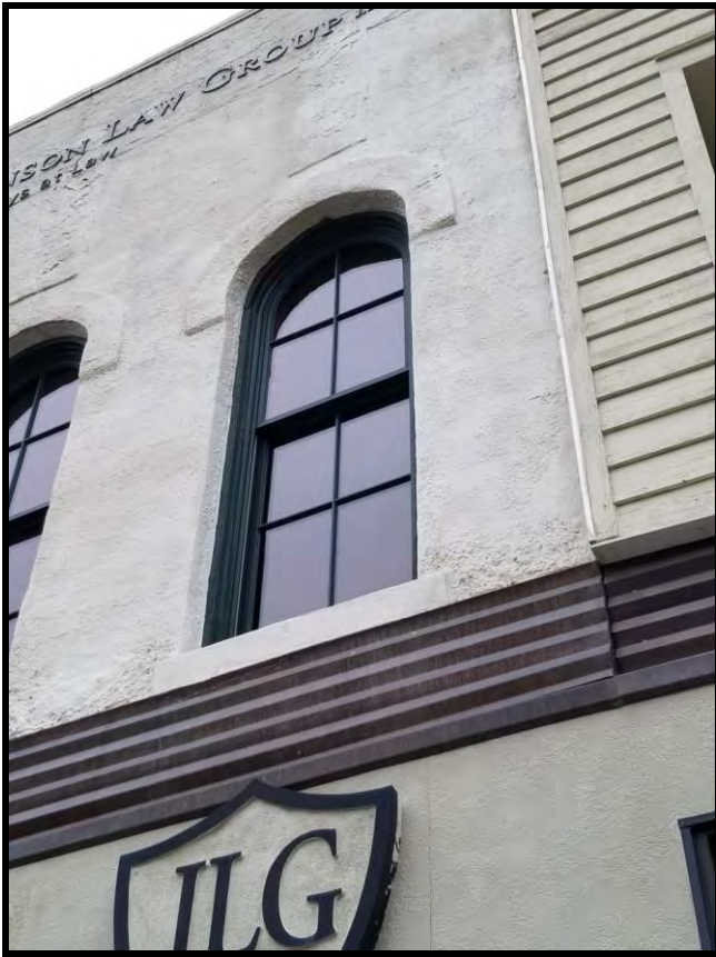
Figure 7 Window at 115 W. Front Street.
