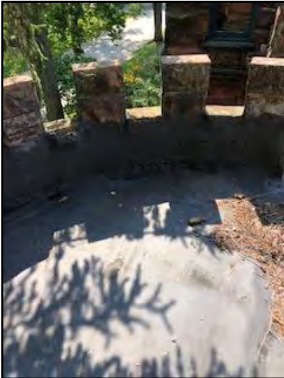
Figure 15 Flat portion of roof.
