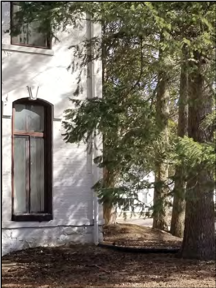
Figure 7 Downspout on southwest corner of house on the front facade.
