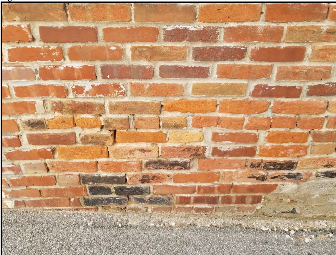
Figure 3 East elevation of the subject property.
