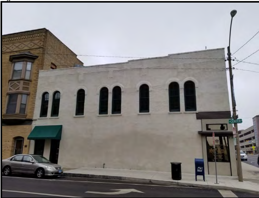
Figure 8 West elevation of 115 W. Front Street.
