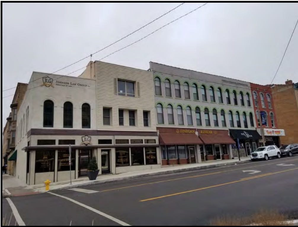
Figure 4 111-115 W. Front Street Streetfront facades
