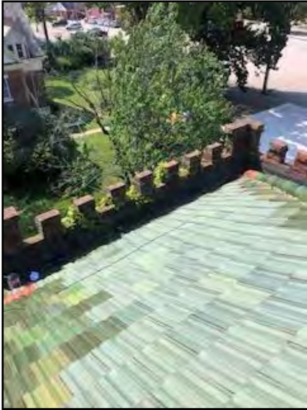
Figure 11 View from top of roof.
