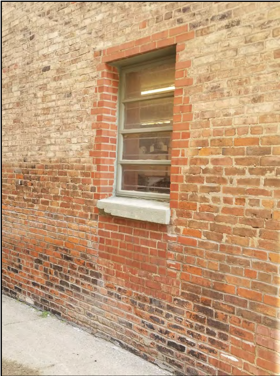
Figure 10 West elevation of subject property showing previous brick replacement.
