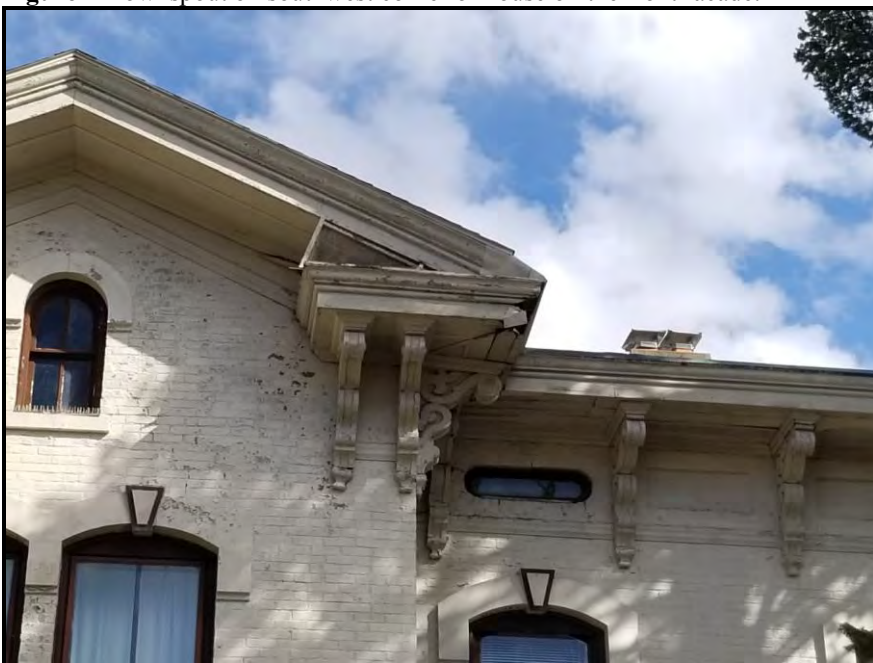
Figure 8 Cornice on front façade showing box gutter.
