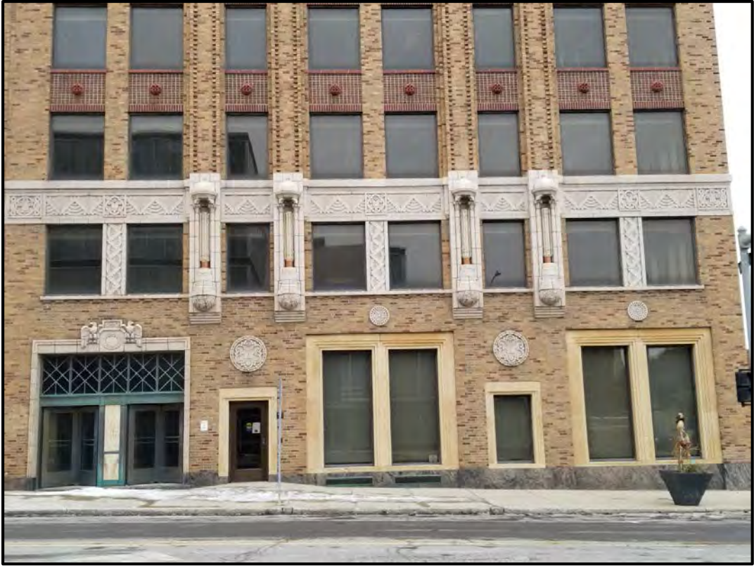
Figure 3 South Entrance of the State Farm Building at 112 E. Washington Street.
