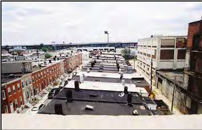
Figure 2 Recommended A cool or green roof is best installed on a flat roof where it cannot be seen from the public right of way and will not negatively impact the character of the historic building.
