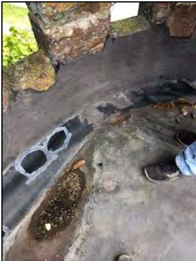
Figure 6 Flat portion of roof.
