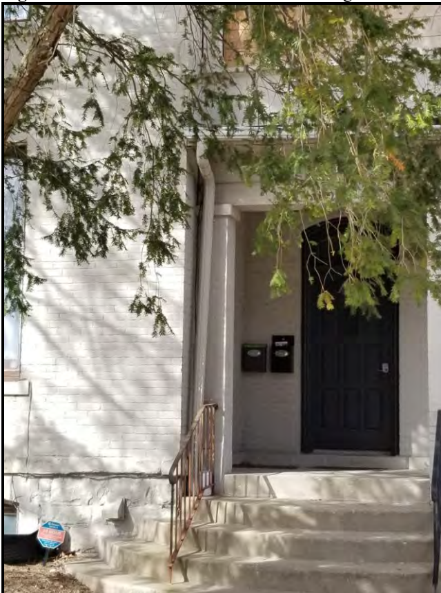
Figure 3 South entrance on rear addition showing downspout - facing E. Chestnut Street.
