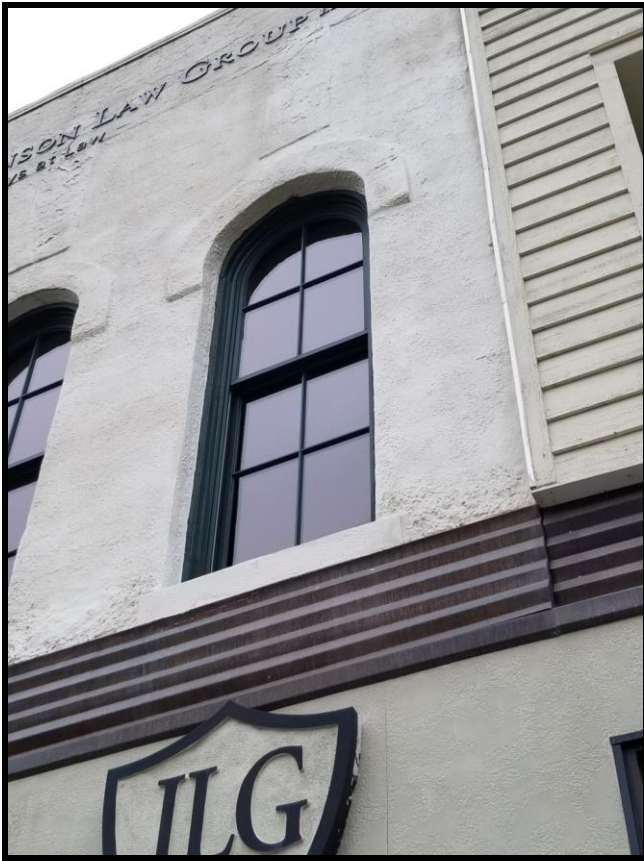
Figure 7 Window at 115 W. Front Street.
