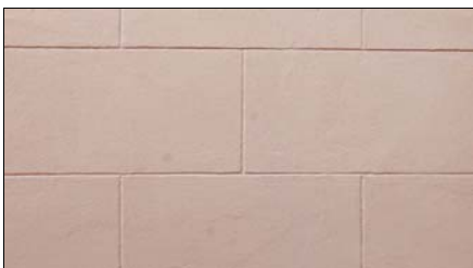
Scored Stucco – Smooth finish with scoring to simulate stone joints.
