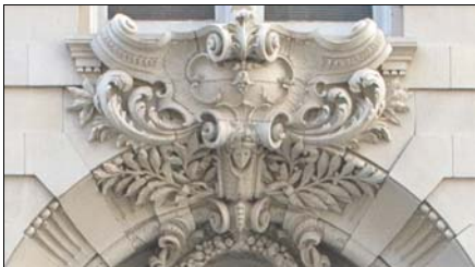
Terra Cotta – Fired-clay, non-structural building components, often with colored glaze, used for decorative, ornate details and wall finishes.
