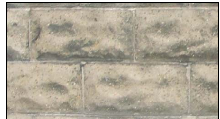
Textured Concrete Block – A structural building material made by mixing water, cement, sand and aggregate, placing it in forms and hardening; commonly used for foundations, walls and piers, popular in the early to mid-20 th century.
