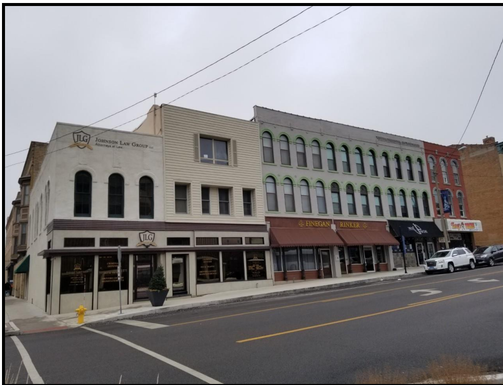
Figure 4 111-115 W. Front Street Streetfront facades
