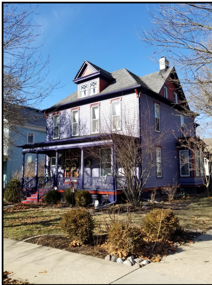
Figure 1 Photo taken 1/16/2020 of the existing roof.
