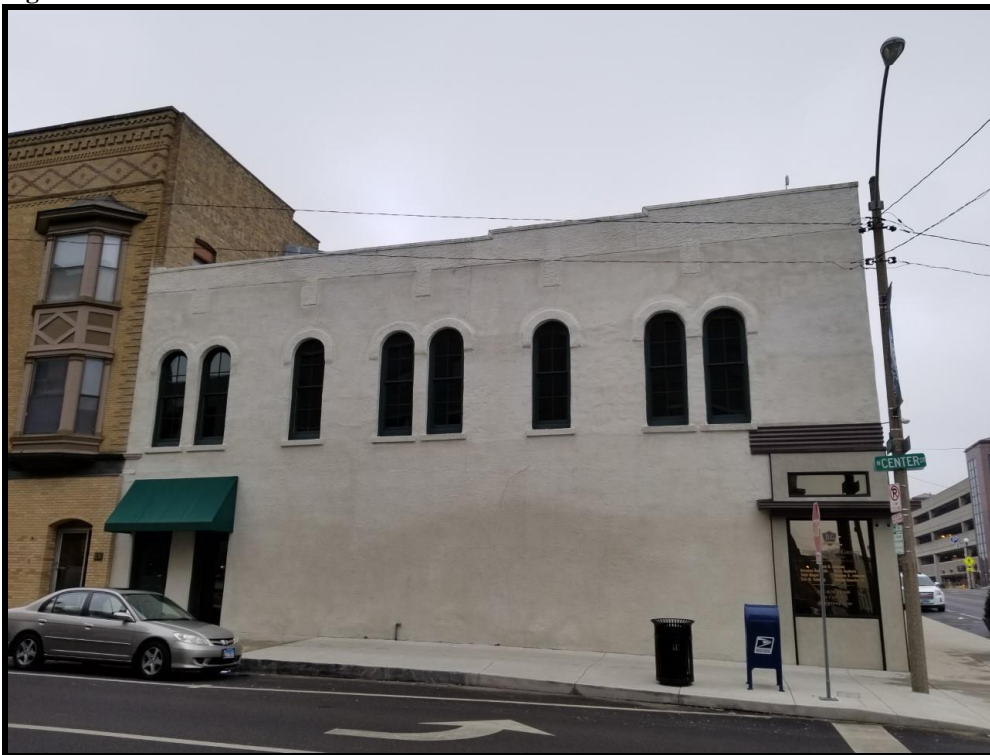
Figure 8 West elevation of 115 W. Front Street.
