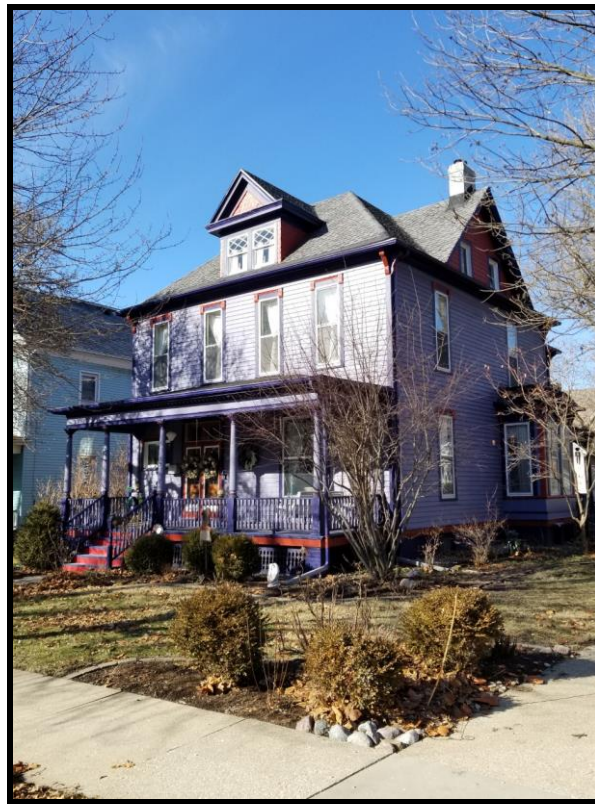
Figure 1 Photo taken 1/16/2020 of the existing roof.
