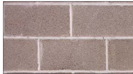
Concrete Block – A structural building material made by mixing water, cement, sand and aggregate, placing the mix in forms and hardening; commonly used for foundations, walls and piers.
