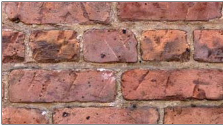
19 th Century Brick – A soft, fired-clay, fairly regularly shaped building component; often with color and surface variations; used primarily in walls, piers, foundations and exterior pavers.
