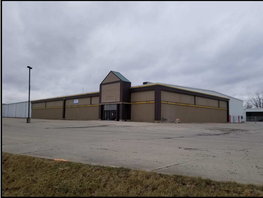
Figure 2 The subject property at 1707 E. Hamilton Road.
