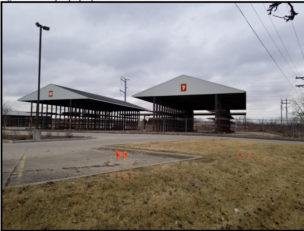
Figure 3 West of the building at 1707 E. Hamilton Road
