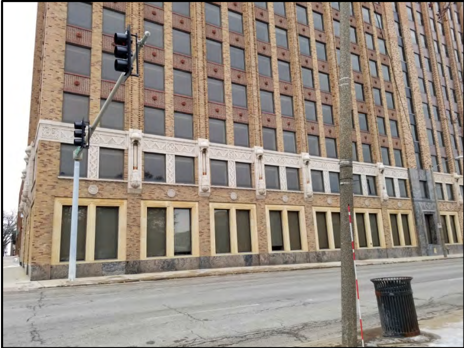
Figure 5 South portion of east elevation.
