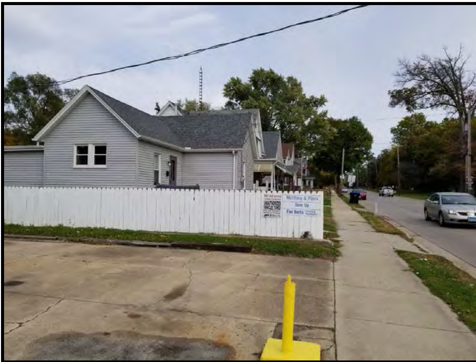
Figure 13 Fence at 929 W. Wood Street fence is finished on both sides.
