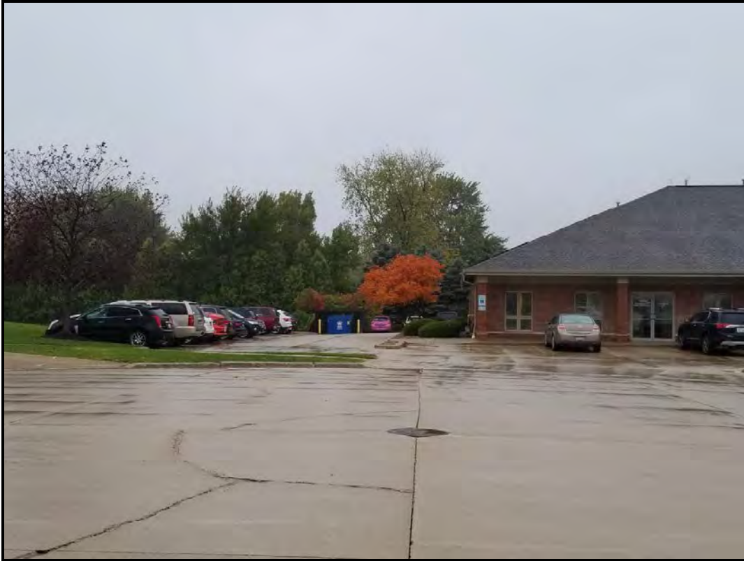
Figure 5 Front and side view of the office.
