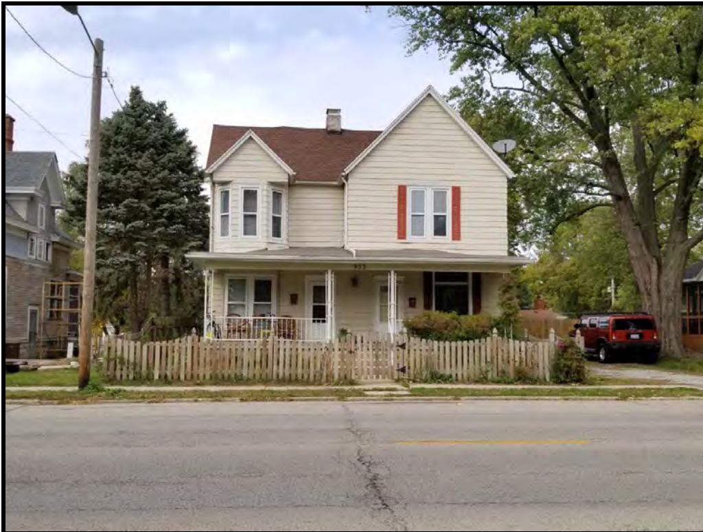
Figure 11 Front yard fence at 923 W. Wood unfinished side faces property owner.
