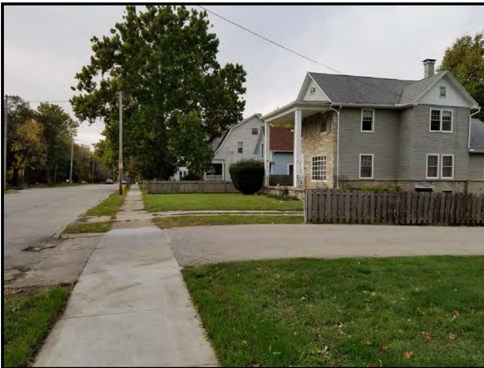
Figure 15 Looking west towards 907 W. Wood Street.
