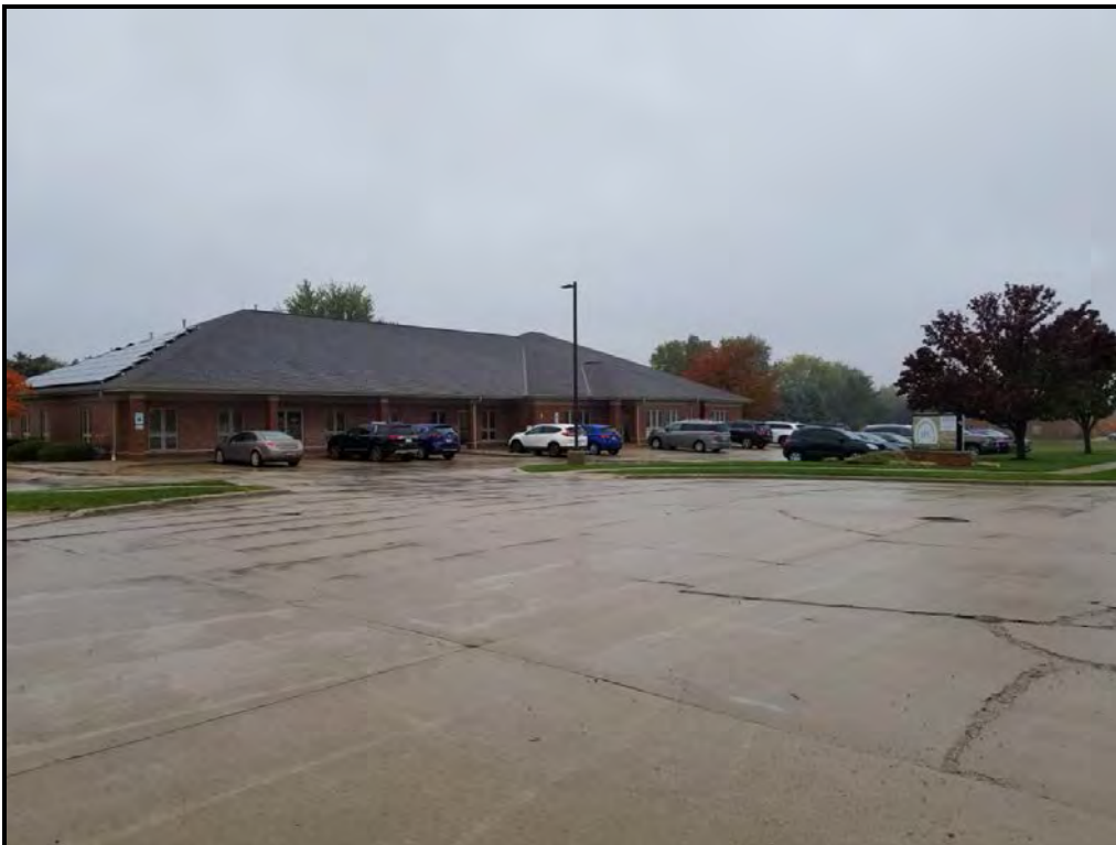
Figure 4 Front view of the office from the cul-de-sac right-of-way.
