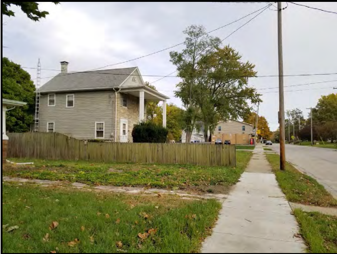
Figure 14 Fence on the west side of 907 W. Wood Street unfinished side faces property owner.
