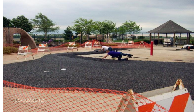
The new surface is installed at McGraw Park sprayground
