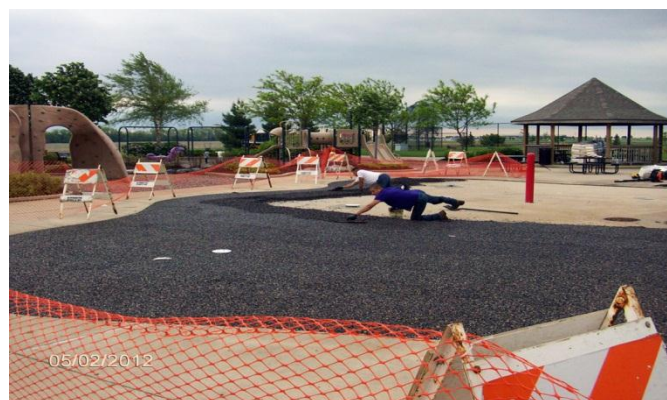
The new surface is installed at McGraw Park sprayground
