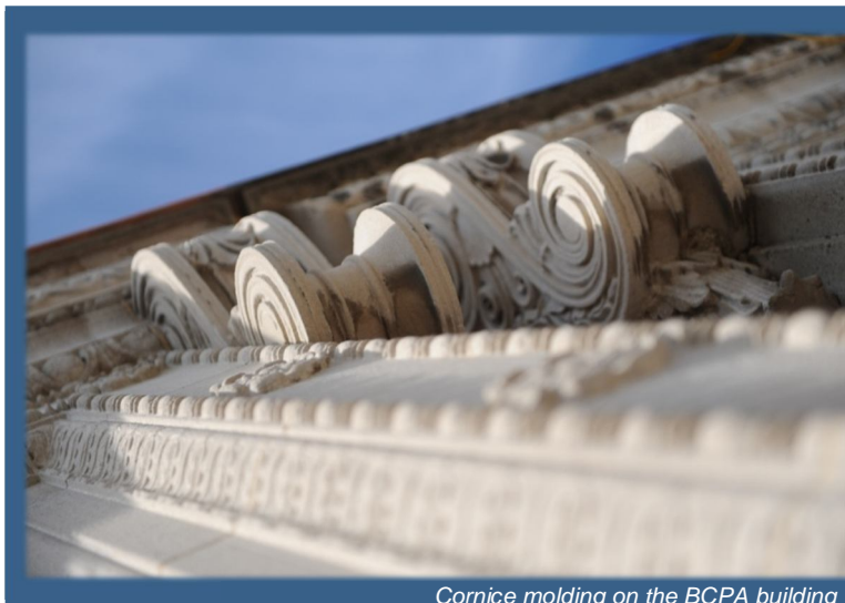
Cornice molding on the BCPA building
