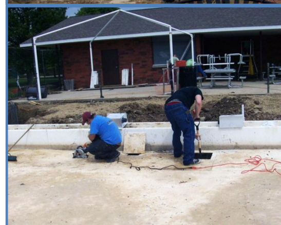
Parks Maintenance works on the balance tank at O'Neil Pool.
