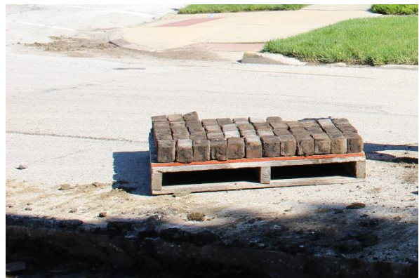
6. Carefully stack undamaged bricks on a pallet. Count on having to discard 30 percent of the bricks because of various types of damage.
