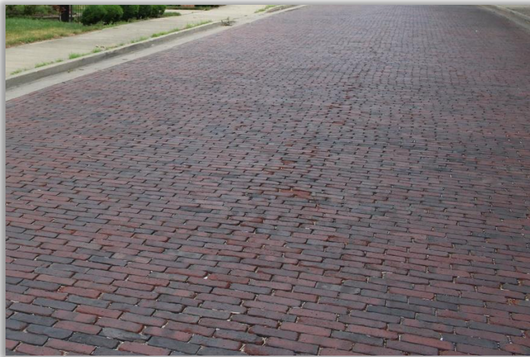
Figure 2: Highest-rated brick street in Bloomington (PASER 10) (Davis Ave., Jefferson St. to Washington St.)
