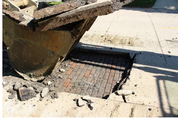
2. Lightly scrape over the asphalt surface. The asphalt will peel away without damaging the bricks, if done correctly. There should be little residual.
