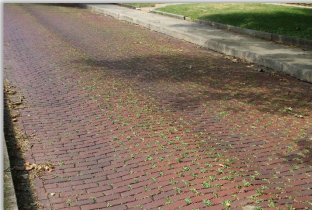
Figure 18: Effects of driving on vegetation between bricks
