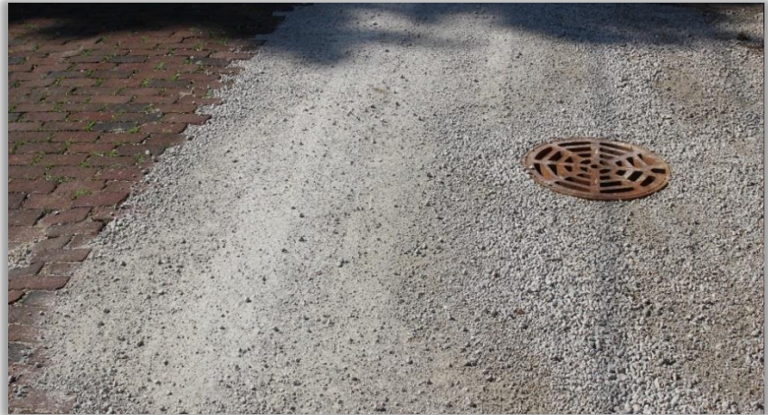
Figure 16: Temporary gravel patch
