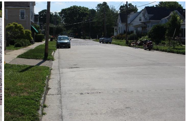
Figure 10: Concrete portion of Chestnut St., from Oak St. to Mason St.
