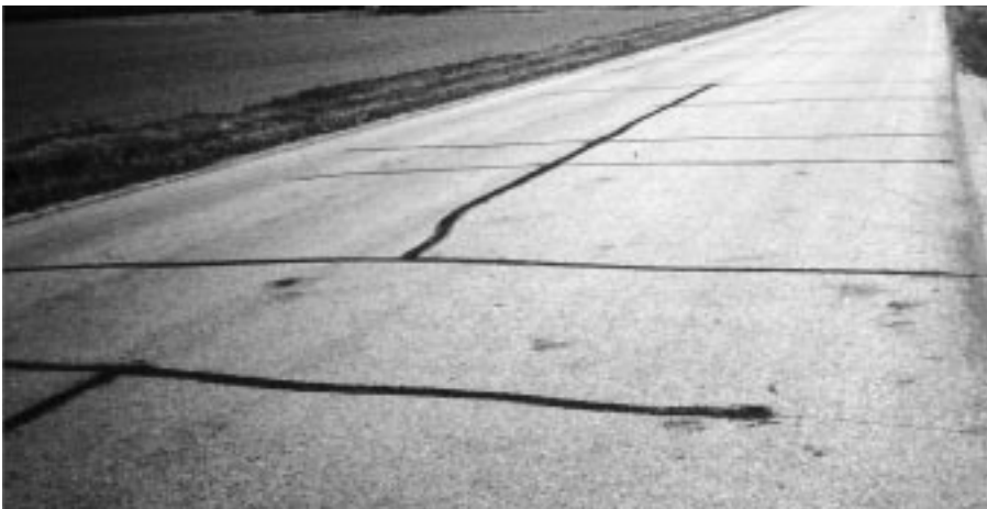
▼ Open crack, 1/2" wide; adjoining pavement sound.
