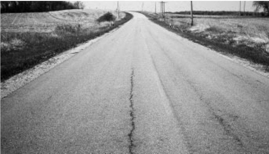
▼ Slight rutting; patch in good condition.
