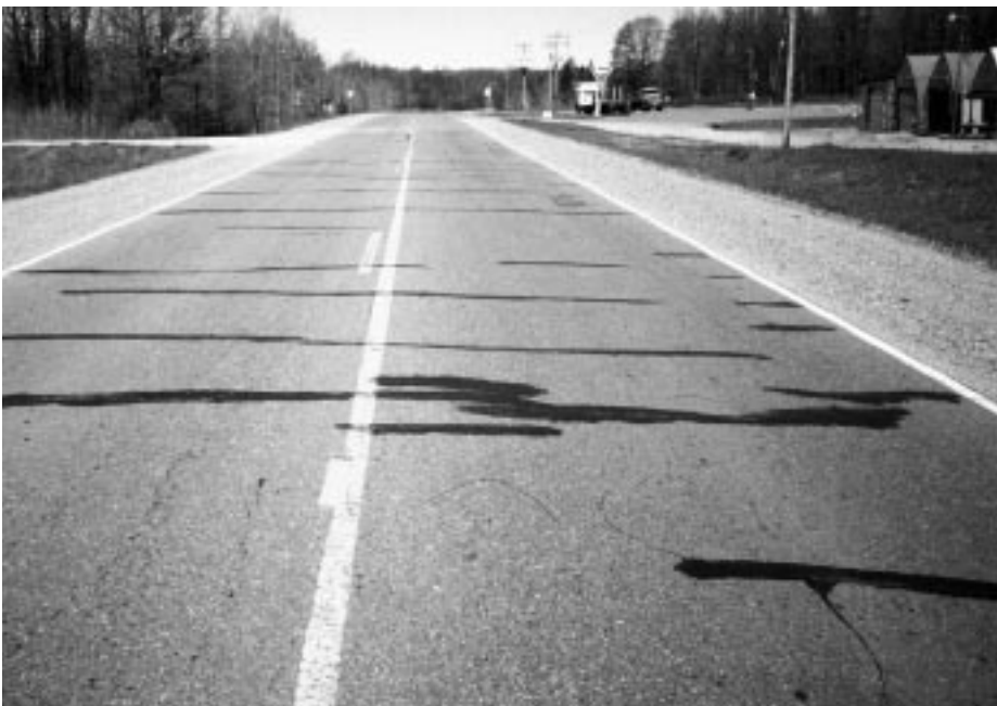
◀ Sealed cracks, a few feet apart.
