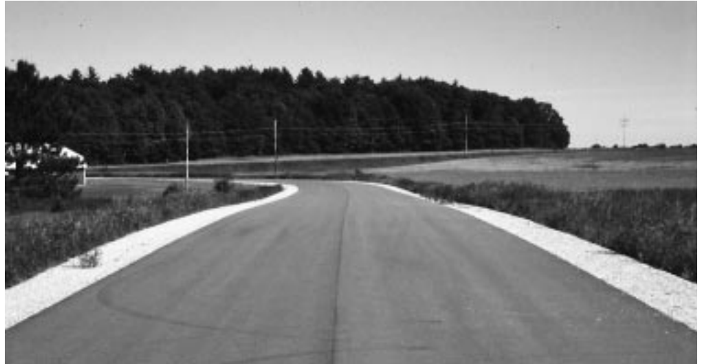
▶ RATING 10 New construction.
