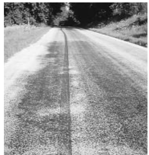
▼ Moderate flushing.
