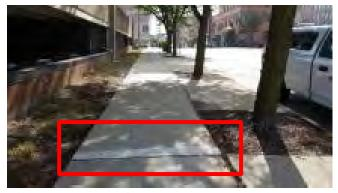
grinding has been a pay item in the regular sidewalk contract, and the pay item is in this year's regular sidewalk contract. However, the City is increasing use of grinding as a way to address sidewalk settlement in certain neighborhoods, primarily on the east side, where concrete is in good physical condition but displacement between adjoining sidewalk panels is common.
