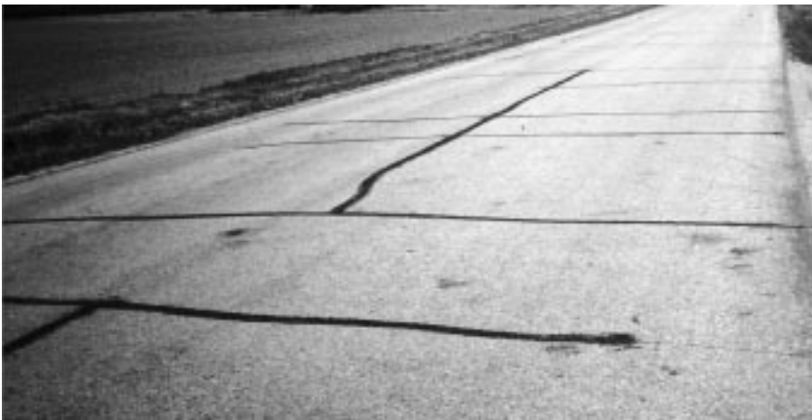
▼ Open crack, 1/2" wide; adjoining pavement sound.
