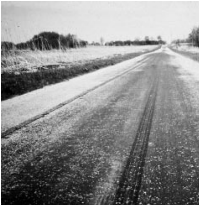
▼ Severe flushing.
