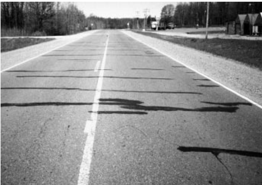
◀ Sealed cracks, a few feet apart.
