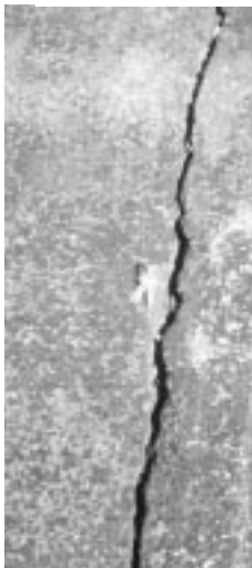
▼ Open crack, 1/2" wide; adjoining pavement sound.
