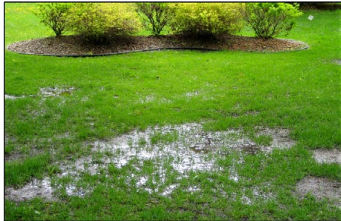
Figure 4. Ponded water over the absorption field is a sign of septic system failure. 16
