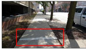
rather than replacing the panel. Major displacements – generally over an inch – are ordinarily rectified with panel replacement, because the cost of the grind begins to approach replacement cost.
