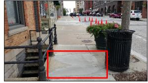
condition of concrete panels remains good, but displacements are present. The City's contractor completed approximately 400 sidewalk grinds at east side locations through early August.
