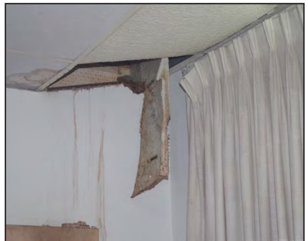
Right: Water damaged and collapsed ceiling tiles in the vacant hospital.
