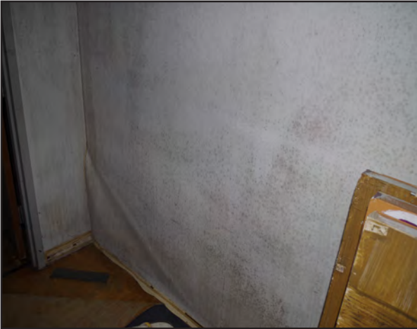
Left: Water damage and mold growth on an interior wall in the vacant hospital.
