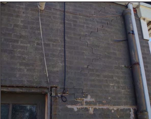
Left: Step cracking on the exterior walls of the former Shell building.
