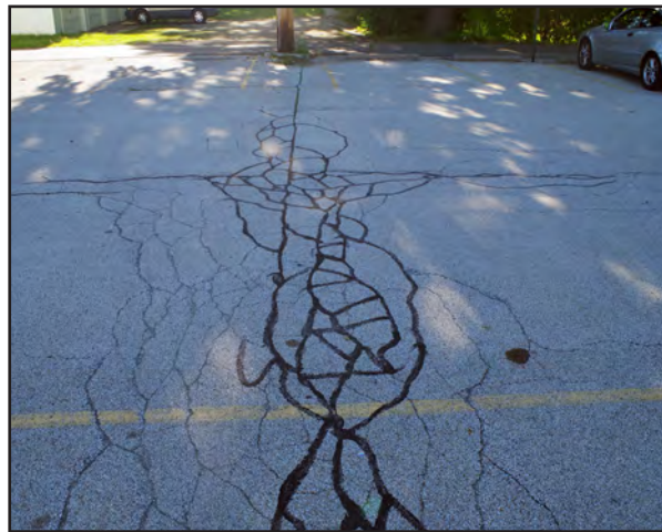
Left & Right: Cracking in the asphalt parking surface at 208 East Chestnut Street.
