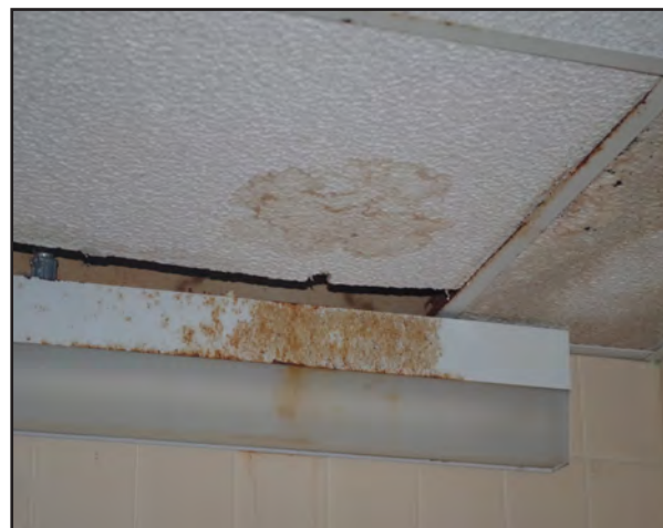
Left: Water running down the wall of the Creativity Center rusted the ceiling structure and stained the wall.
