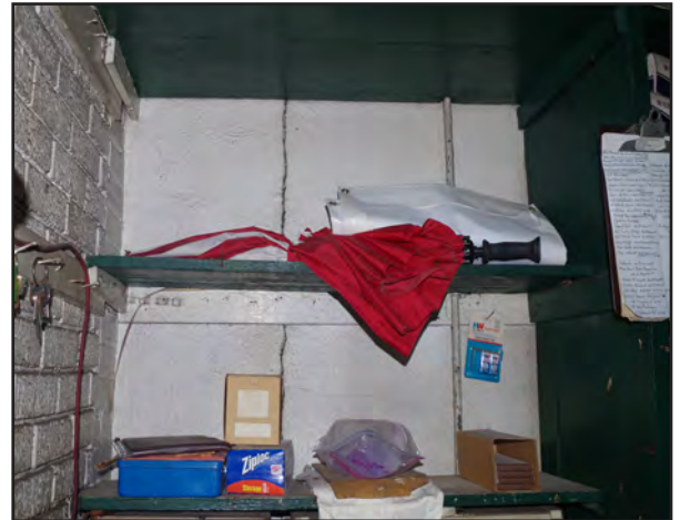
Left: Step cracking and shifting of the concrete blocks on the interior wall of the former Shell.
