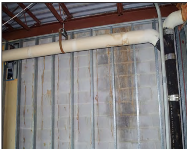
Left: Water running down the wall of the Creativity Center rusted the ceiling structure and stained the wall.
