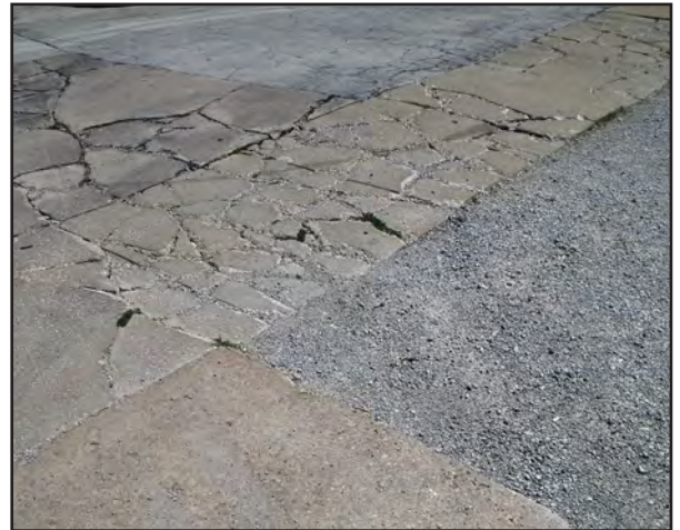
Left: The edge of the pavement along West Walnut Street is deteriorated. (Between North Main Street and North East Street)
