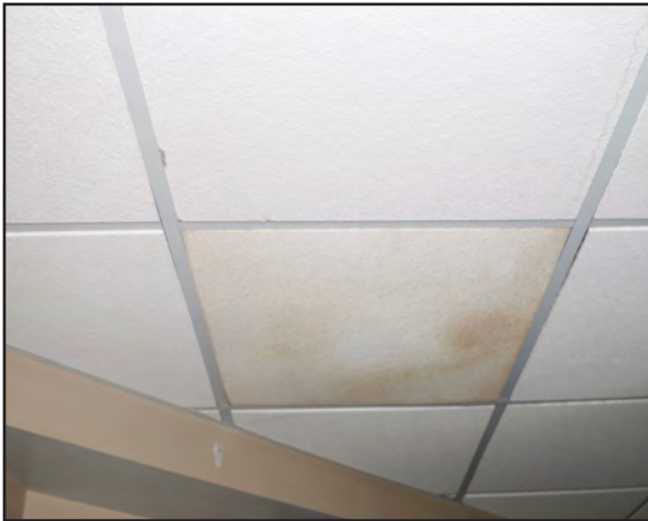
Left & Right: Water damaged ceiling tiles on the interior of the former dormitory.
