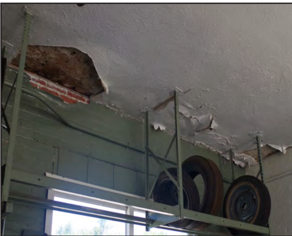
Left & Right: Water damage to the ceiling of the former Shell building.
