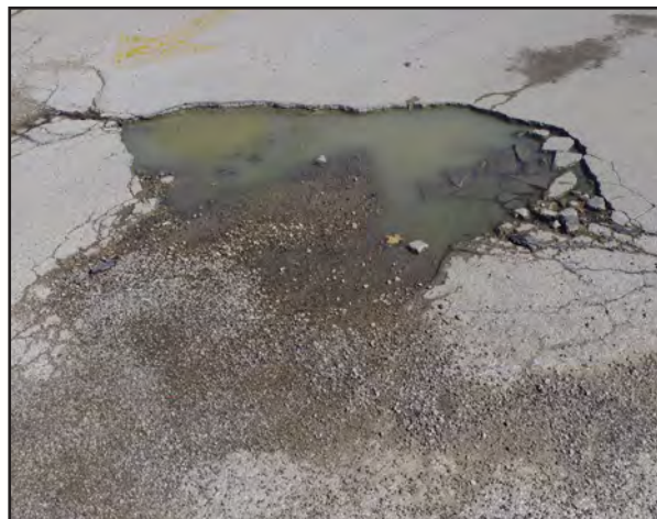
Left: Cracking in the asphalt parking lot located at 103 West Chestnut Street.
