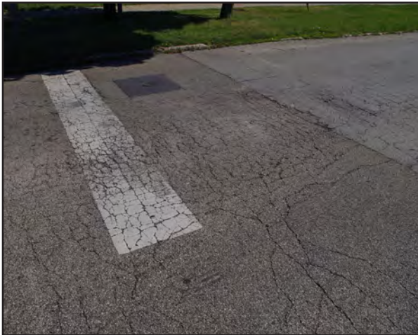
Left: The paving at the intersection of North Main Street and West Chestnut Streets has alligator cracking.
