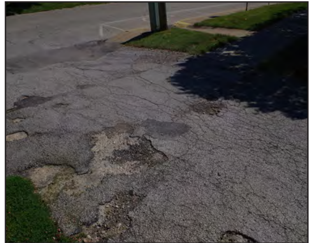
Left: The paving at the intersection of North Main Street and West Chestnut Streets has alligator cracking.
