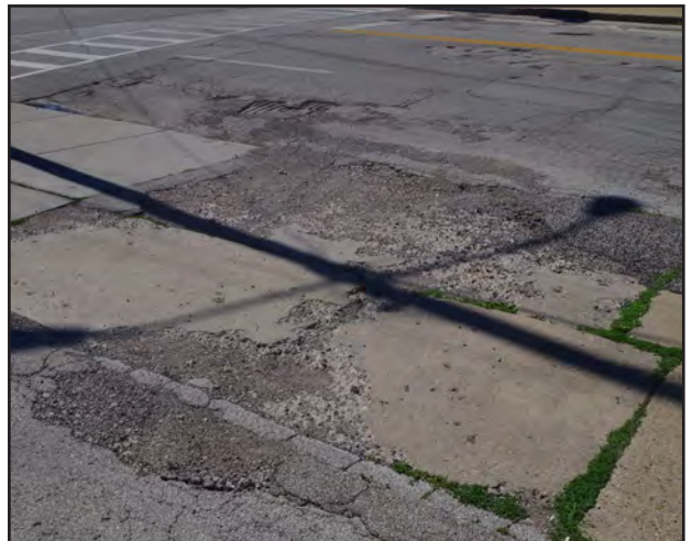
Left: The pavement on West Chestnut is cracked and deteriorated. (Between North Main and North East Streets)
