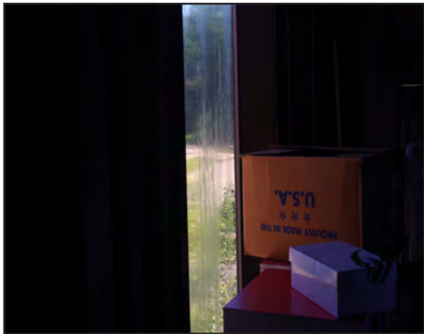
Left: Moisture in a window, due to failed seals, in the Creativity Center.
