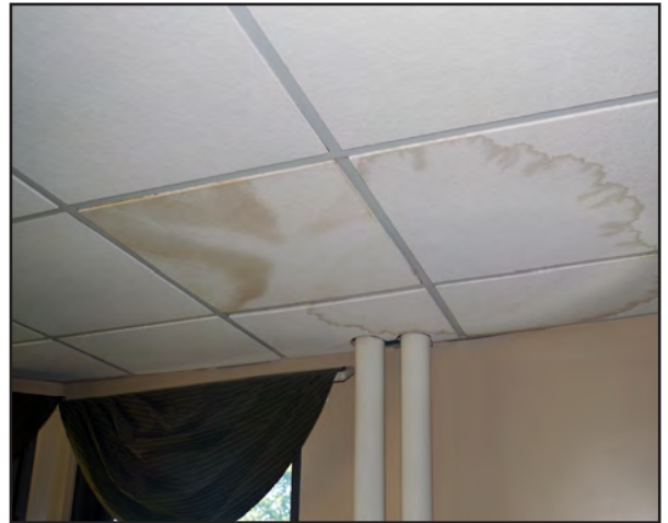
Left & Right: Water damaged ceiling tiles on the interior of the former dormitory.
