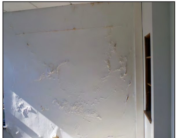
Left & Right: Water damage to the interior walls on the vacant dormitory.
