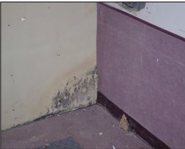
Left: Mold growth on an interior wall in the vacant hospital building.
