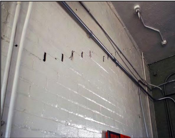
Left: Step cracking and shifting of the concrete blocks on the interior wall of the former Shell.
