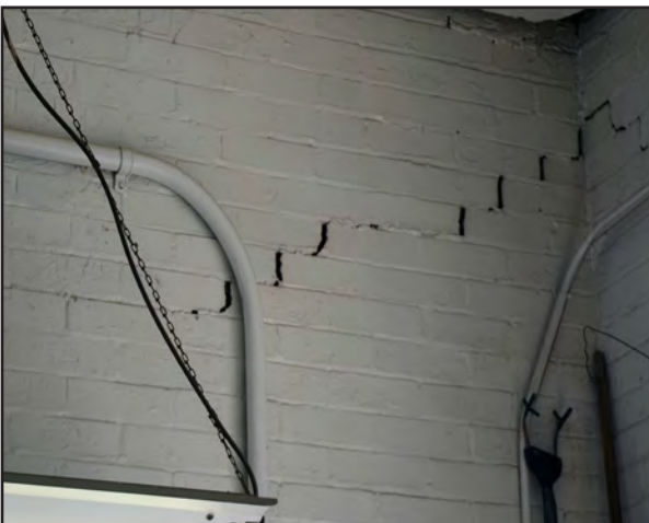
Left: Step cracking and shifting of the concrete blocks on the interior wall of the former Shell.
