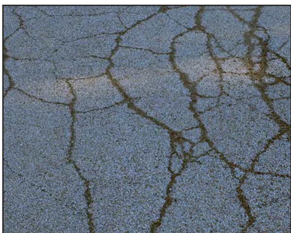
Left & Right: Cracking in the asphalt parking surface at 208 East Chestnut Street.
