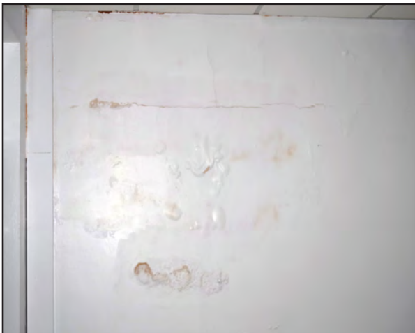
Left & Right: Water damage to the interior walls on the vacant dormitory.
