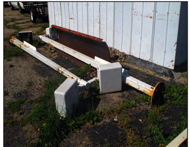
Right: The lighting standards for 802 North Main Street are rusted and lying on the ground.
