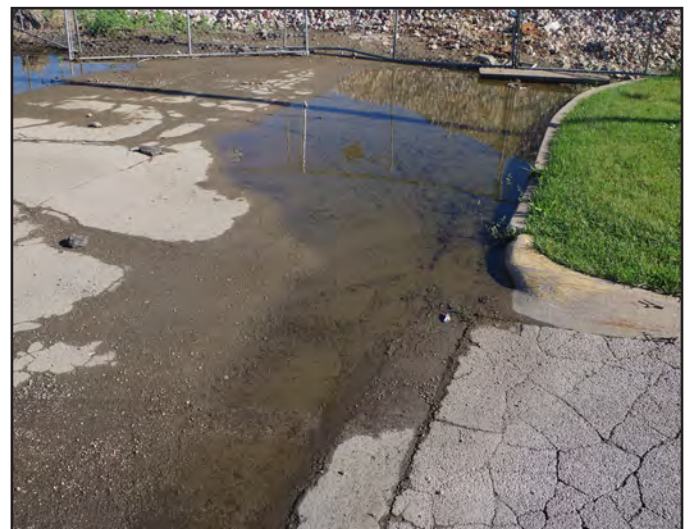
Standing water on the vacated North East Street right-of-way.
