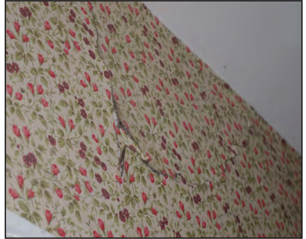
Right: Cracking on the interior plaster wall of the Burr House.
