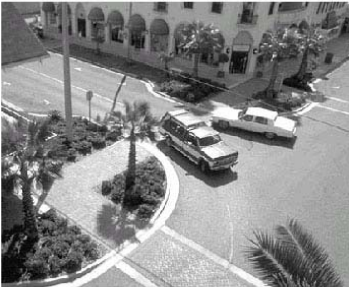
This curb extension in Venice, Florida reduced motorists turning speeds by 6-8 MPH. Pedestrian crossing distance and time exposed to traffic was also reduced.
