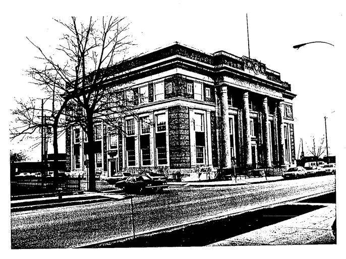
The John B. McBarnes Memorial Building is a three story masonry structure of Neo-Classic design. It has a full basement whose walls are all made of hand fired red brick. The walls above are hollow glazed tile faced with pale yellowish tan brick probably from St. Louis. It is trimmed with Bedford limestone. The floors are of wooden construction, covered with terrazo in many locations.
