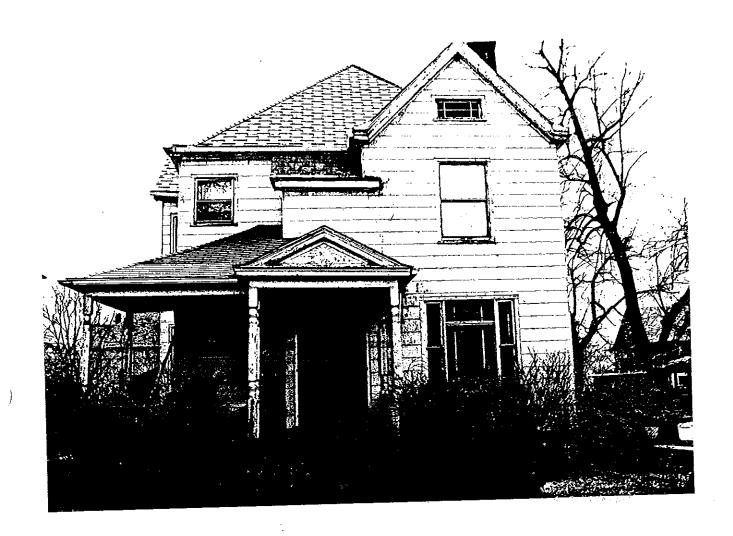
The Charity Adams house is a large two story frame house built on an irregular plan, in a Queen Anne style. Application of asbestos siding c 1950 destroyed much of its detailing.
