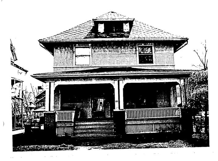
The H.W. Kelley house is a two story clapboard frame structure. It is built upon the American four square plan, a popular layout for this type of Arts and Crafts design house. The house is in good condition.
