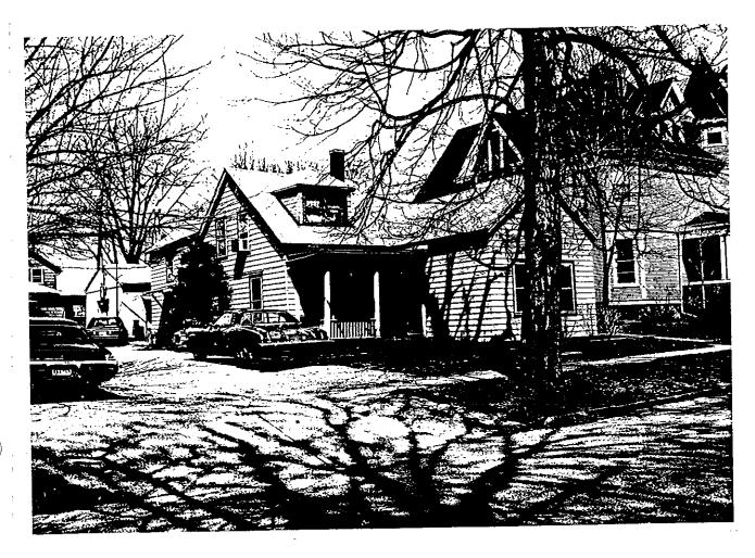
The Prince/Mower house, the east half of which dates c 1855, is a frame structure of parallel rectangles in plan. It had gained its present form by 1901 although shingle siding was applied to it later in this century.
