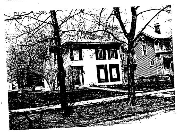
The William T. Wood house is a two story frame structure originally Italianate in design. It is presently covered with stucco, applied c 1950.
