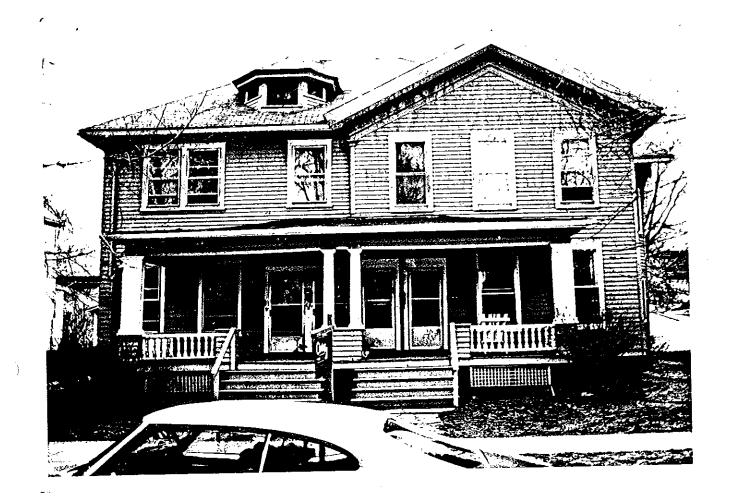
The Young/Perrigo house is a New England side hall type house similar to 510 E. Grove which was enlarged to a multi-family structure by an addition designed by a local architect. This clapboard sided structure was originally intended to be a duplex but is now in four or more units. Structurally it appears to be in good condition.
