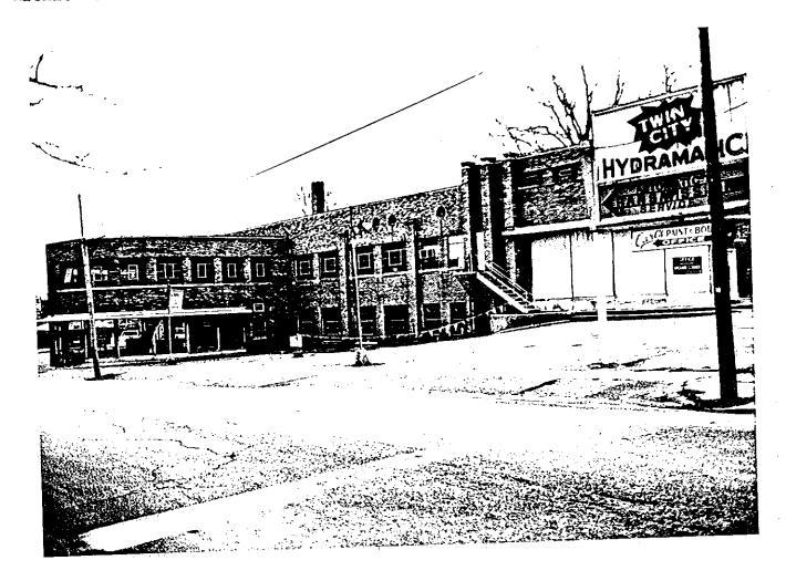
The Thornton Motor Company building is a two story masonry structure built in Moderne style as a sales and repair facility for Lincoln-Mercury automobiles. It is an "L" shaped building oriented North-South. The wing which completes the "L" was built in 1949.
