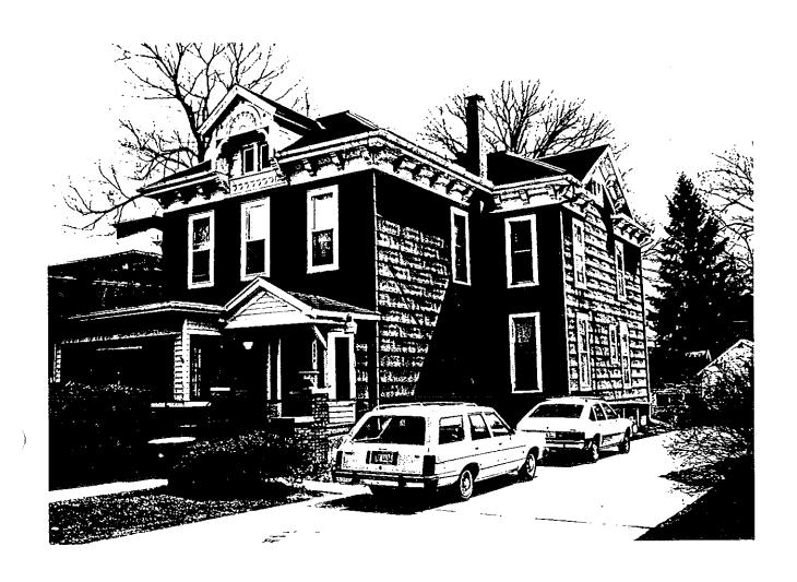
The George Brand house is a two story frame house layed out in an Italianate plan but detailed with Eastlake inspired features. Green asbestos siding and modern porches detract from its original appearance.
