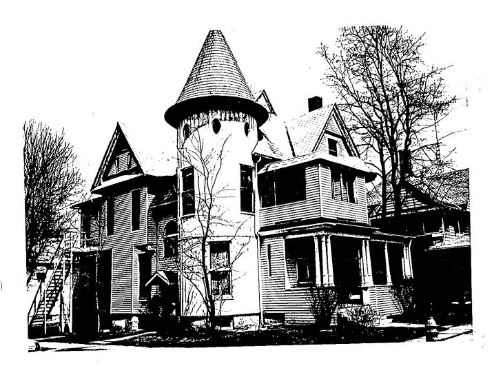
The Augustus Elbe house is a large two story frame structure designed in the Queen Anne style. Its wall surfaces and window and door mouldings have been covered with aluminum siding.
