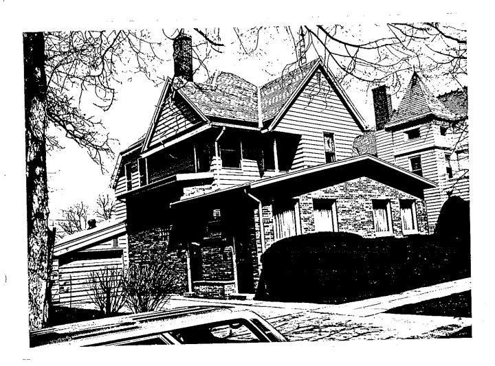
The First M.E. Parsonage is a two story frame structure so severely altered from its originally designed appearance that it barely falls into the purpose of this survey. It should suffice to say that of the house George Miller designed only the roof line remains. The structure cost \$3,500 to build and was used as a parsonage for the First Methodist Church. Frank Crane, the widely published inspirational writer, lived here when preaching in Bloomington.
