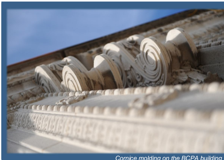
Cornice molding on the BCPA building
