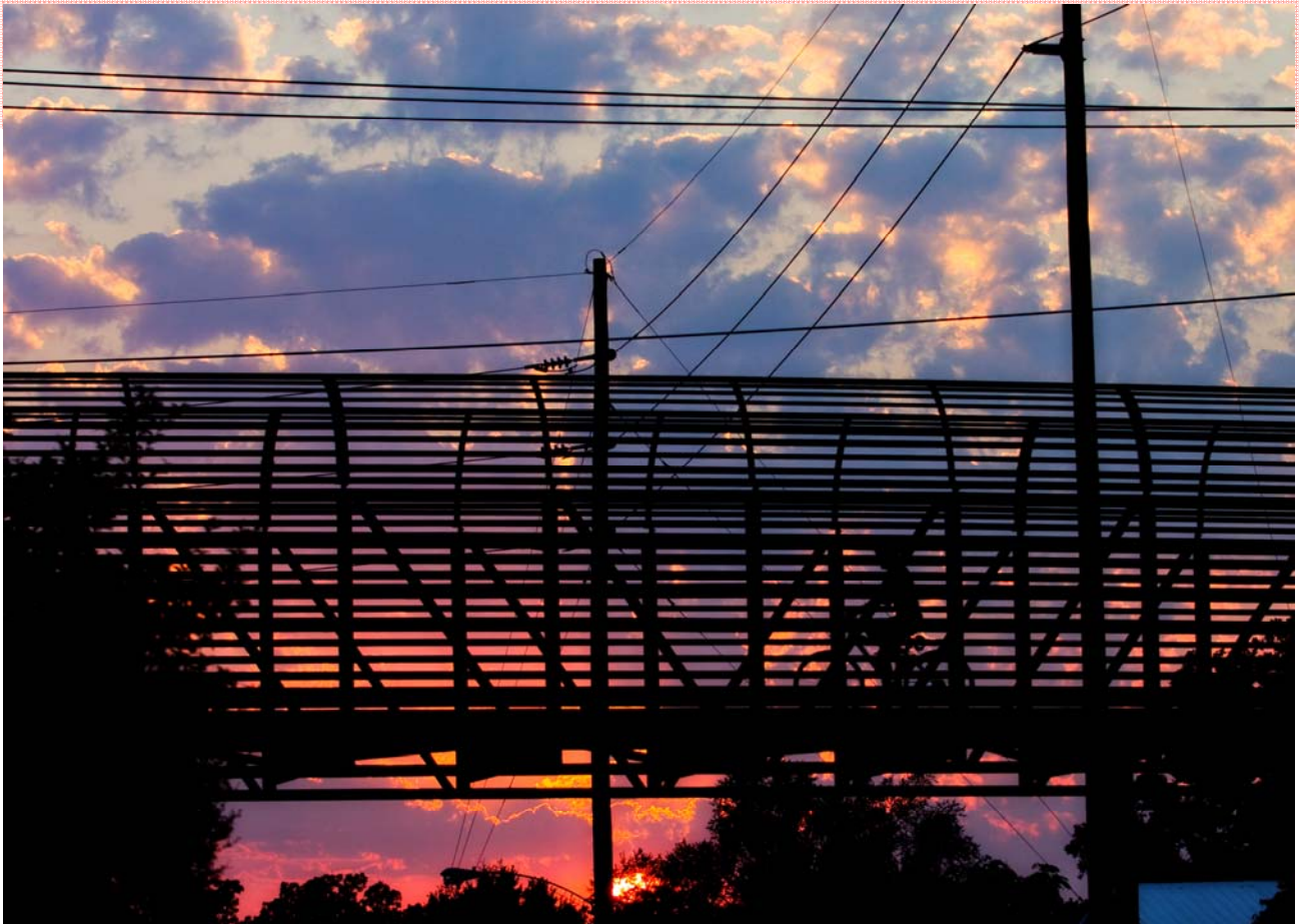
Bridge over Oakland Ave for Constitution Trail, September 2011
