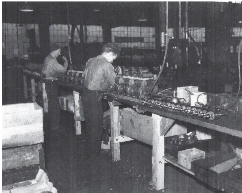
Workers manufacturing the “Oil-O-Matic” in the Williams Factory Building. (Courtesy of the McClean County History Museum)
