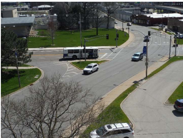
Project south end, Main at Olive, Bloomington
