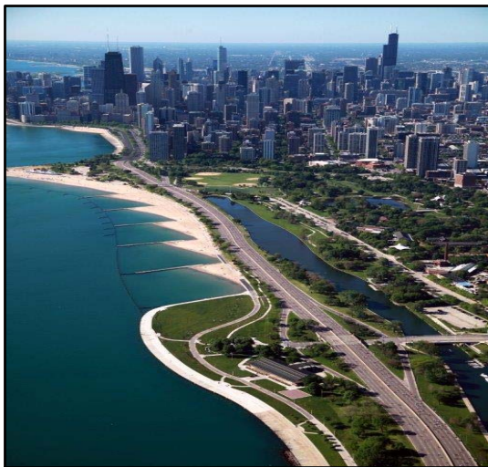
NORTH LAKE SHORE DRIVE IN CHICAGO
