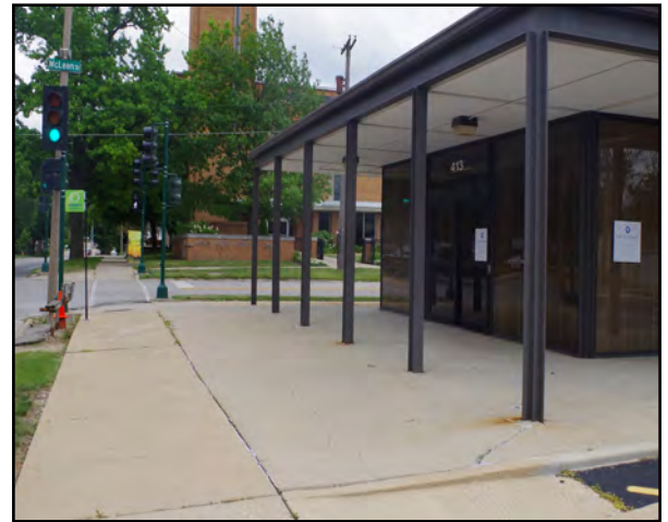
Right: The entire parcel, containing the bank building, has been paved.
