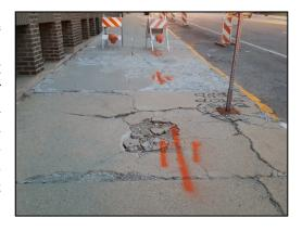
Earlier this year, Connect Transit set up a bus stop along the sidewalk. Complaints soon followed. An inspection by the Engineering Division revealed that the sidewalk, already in poor condition, had rapidly deteriorated in the past year. Public Works closed the sidewalk and the bus stop had to be relocated. Temporary patching options were examined but staff concluded that the damage is too extensive to make patching practical.
