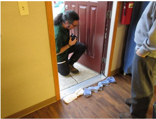
Checking door seal and threshold.
