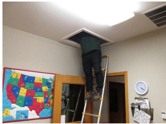
Checking attic insulation levels.
