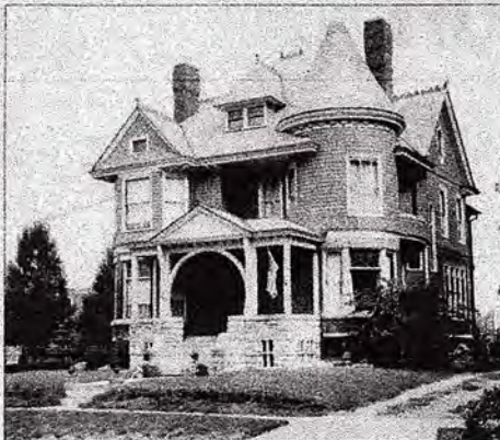
The Oscar Mardel home, relocated to 402 E. Grove, has regained much of its lost grandeur as Diana Krieger and Dawn Peters restore the old house.
