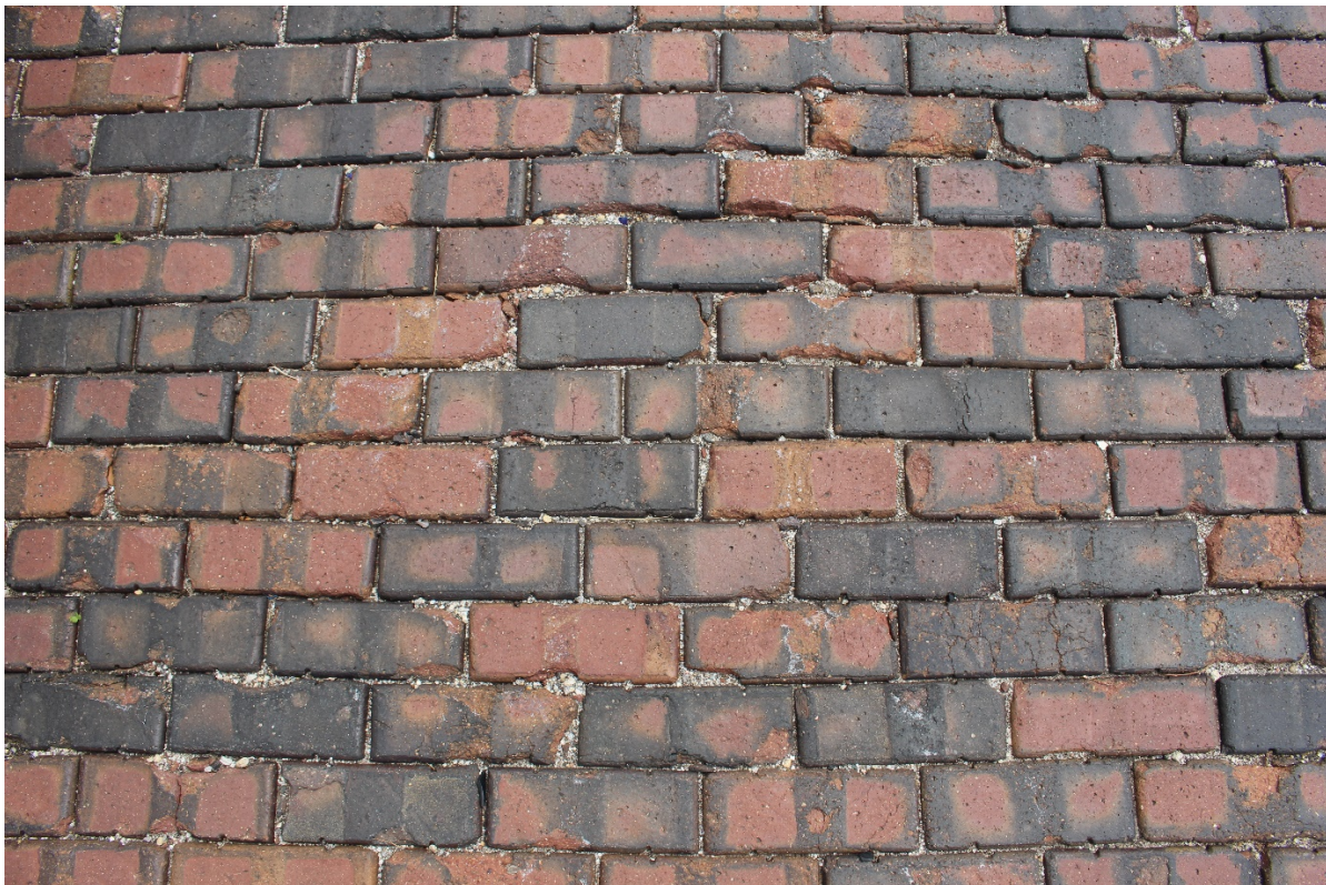
Figure 31: Close-up of brick pavement on Chestnut St., Oak St. to Mason St.
