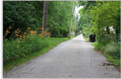
Figure 28: Alley driveway access
