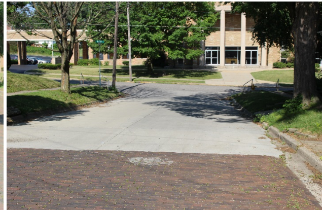
Figure 8: Concrete portion of Elm St., from Center St. to Madison St.
