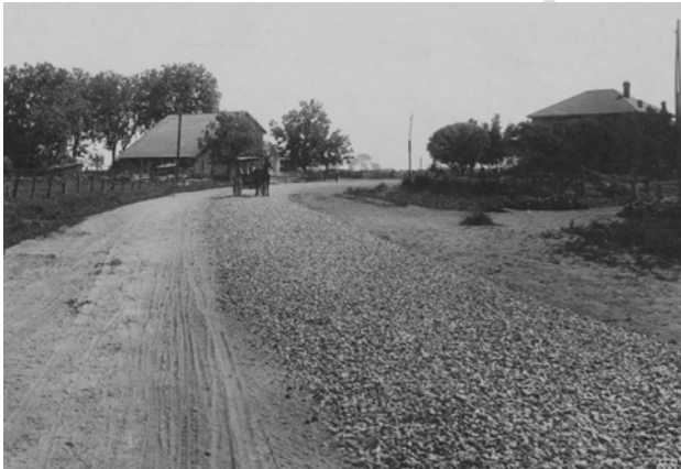
Figure 2: Example of old macadam pavement 1
