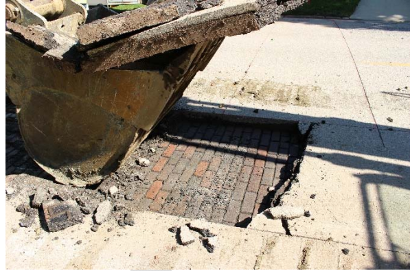
2. Lightly scrape over the asphalt surface. The asphalt will peel away without damaging the bricks, if done correctly. There should be little residual.
