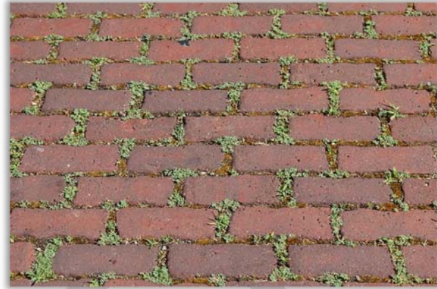
Figure 25: Vegetation between bricks (White Pl.)
