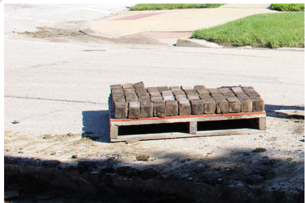
6. Carefully stack undamaged bricks on a pallet on location or at another location, depending on the method used. Count on having to discard 30 percent of the bricks because of various types of damage.
