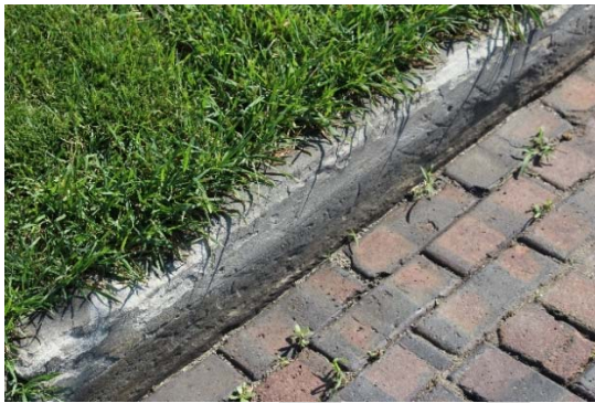
Figure 30: Sandstone curb
