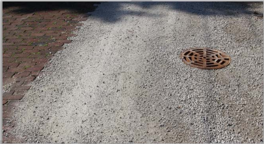
Figure 23: Temporary gravel patch
