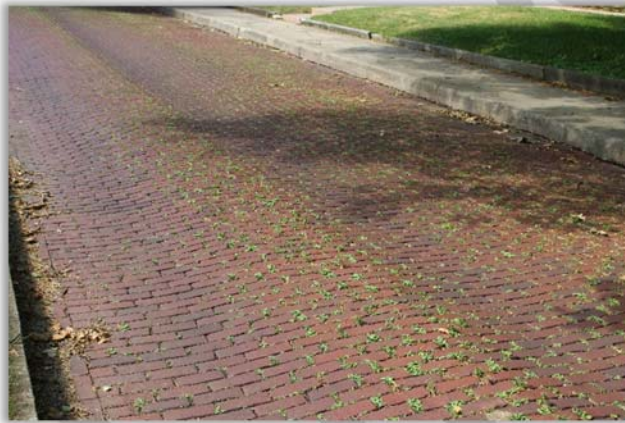
Figure 26: Effects of driving on vegetation between bricks (White Pl.)
