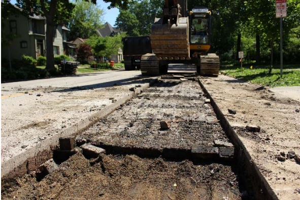
1. This process requires a backhoe with teeth in good condition.
