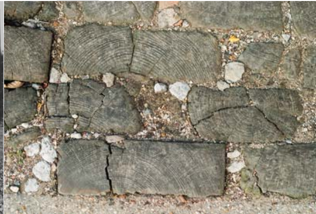
Figure 3: Example of old Nicholson block pavement 2
