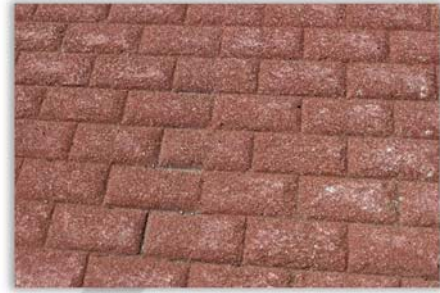
Figure 20: Brick-stamped concrete
