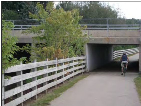
Figure 4.8. Trail underpass of Hershey Road.
