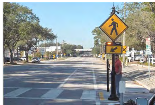
Figure 4.7. Left – median refuge island (courtesy Pedestrian Bicycle Information Center). Right – Rapid Rectangular Flashing Beacon (courtesy FHWA).
