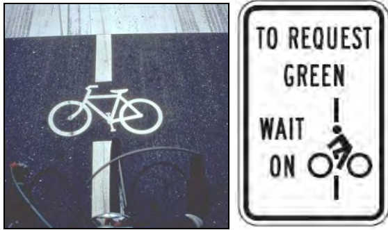
Figure 2.12. Signal activation marking and sign.
