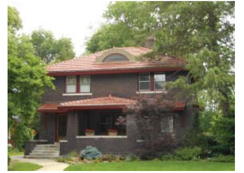
Historic home in Whites Place historic district
