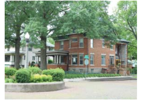
Historic home in Whites Place historic district
