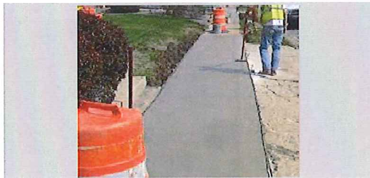
Sidewalk repair being completed.
