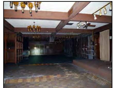
Below: The interior wood floor of the former Elks lodge is buckling.
