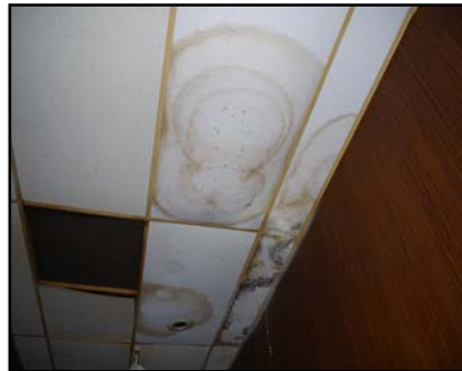
Above: Mold and evidence of water damage on the interior of the former Elks Lodge Building.
