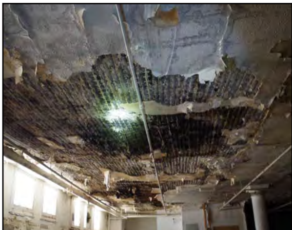
Left & Right: Water damage to the interior of the Front N Center Building has led to the plaster ceiling collapsing. (Lower Level)
