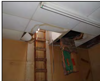
Below: Water damage around the roof access of the former Elks Lodge.
