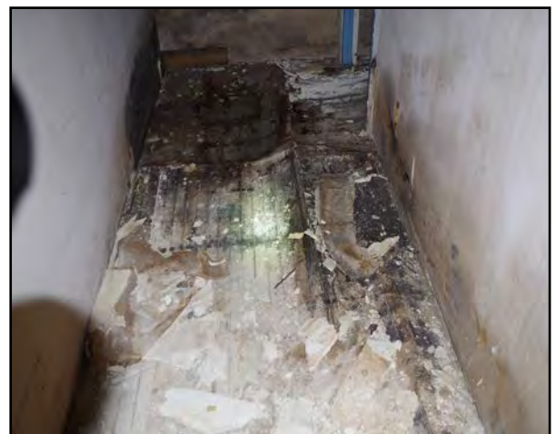
Left & Right: The wood floor in the Front N Center building is buckling. (1st Floor)
