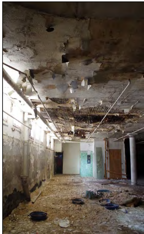
Left & Right: Water damage to the interior of the Front N Center Building has led to the plaster ceiling collapsing. (Lower Level)
