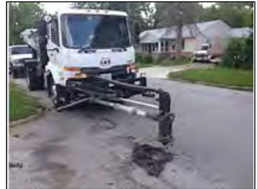
Example of pothole spray injection equipment
